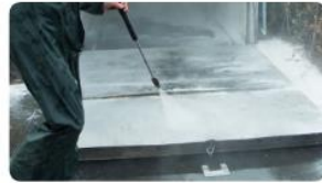
STEP 3 Rinse with water High pressure cleaner (50-150 bar, 12-30L/min.) and let dry.
