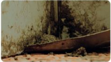
STEP 1 Dry cleaning Take away all rests of manure.
